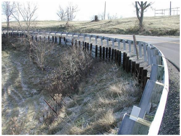
Roadbeds on shale, like this in the Preacherville Formation of the Outer Bluegrass in Bath County, often require additional support on slopes. Photo by Dan Carey, Kentucky Geological Survey.
